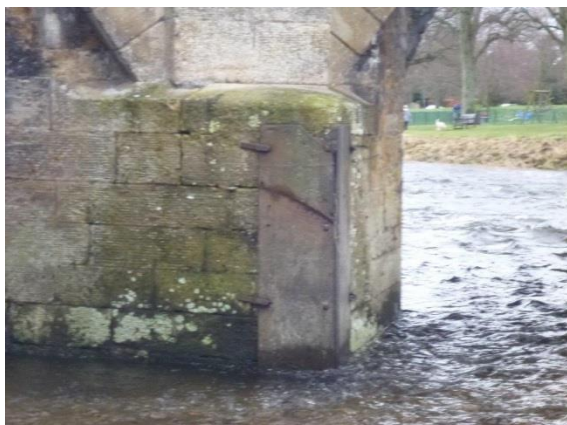
Scour protection on front on pier
