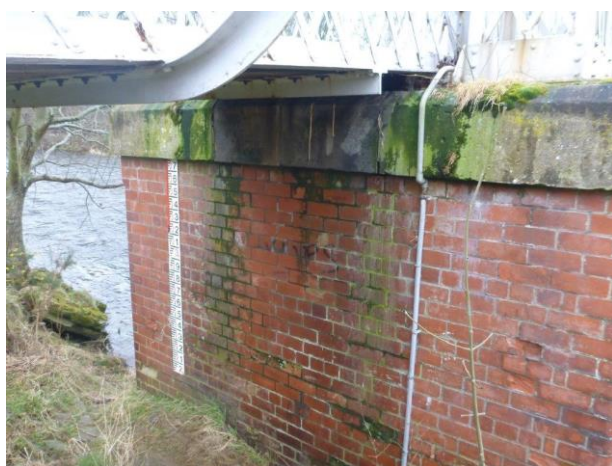
Minor spalling in brickwork and some vegetation growing through cracks in concrete
