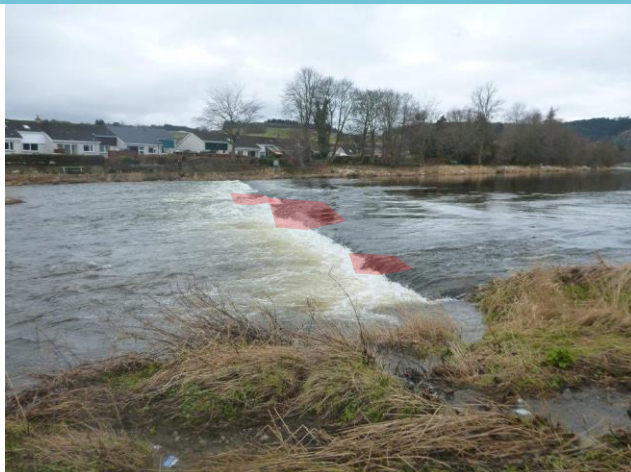
Concrete weir with defects highlighted in red
