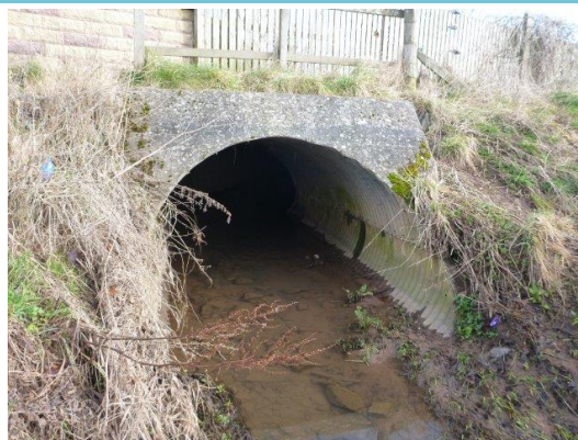
Blockage of diversion channel culvert
