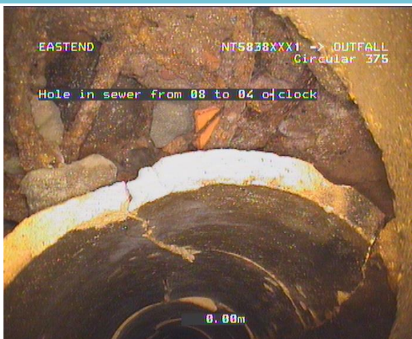
Collapsed roof in culvert
