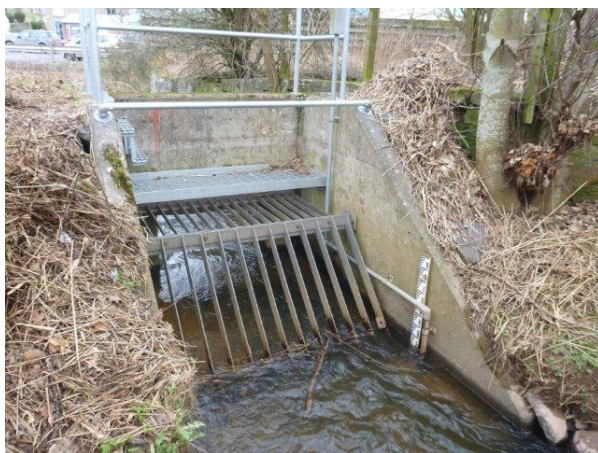
Debris Screen and concrete orifice
