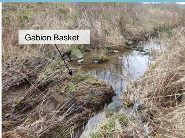
Gabion basket and build-up of silt at entrance to diverted channel
