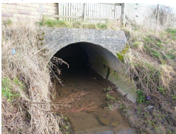
Culvert outlet with concrete headwall
