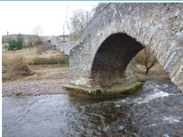
Scour protection on central pier
