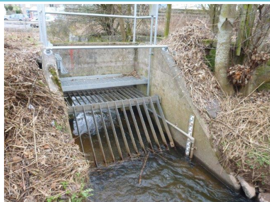
Diversion channel flow control screen
